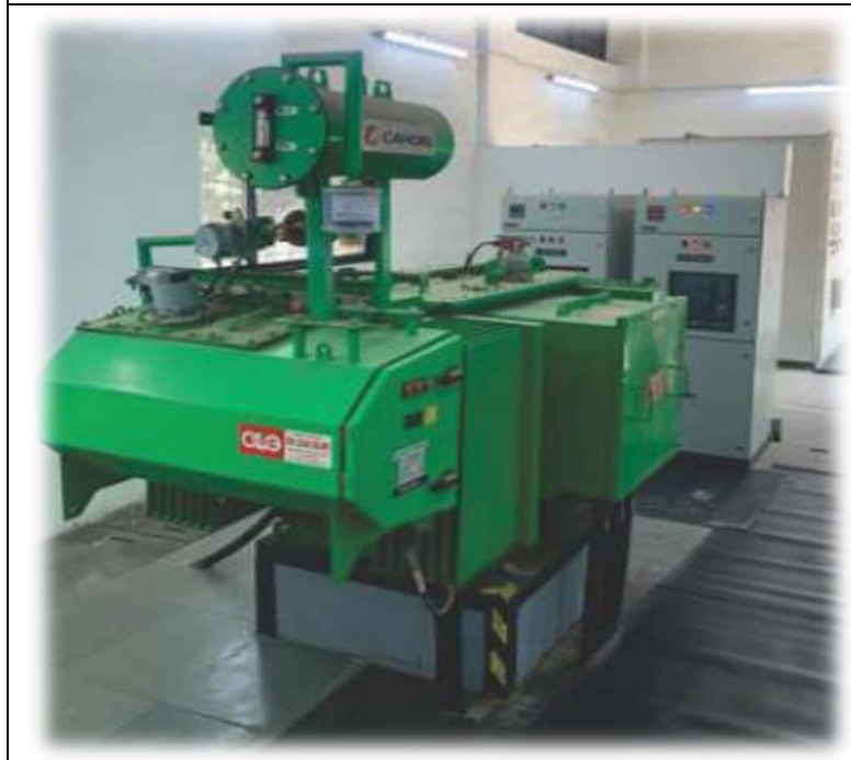
HT Sub Station Works - M/s. Mastek Ltd - Mahape - Navi Mumbai
